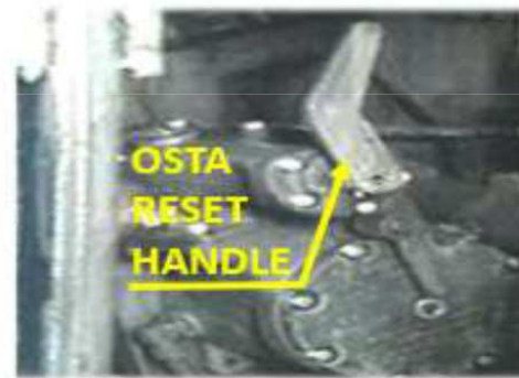
Reset handle in set condition
